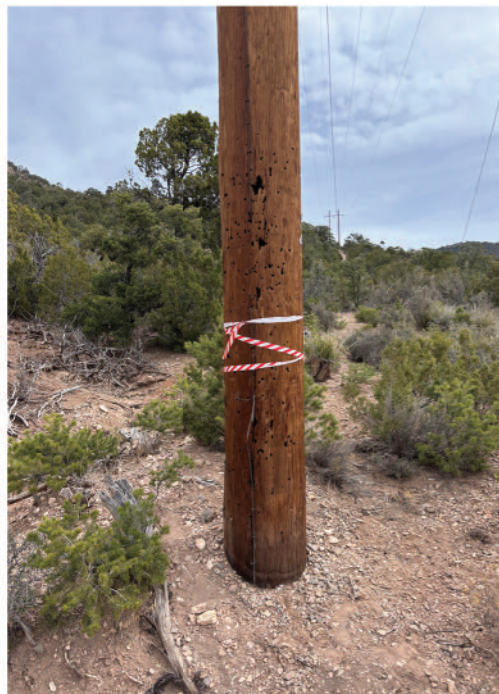
A damaged power pole, shown left with gunshot holes, has been stabilized with a 35-foot pole, right, until weather and conditions allow crews to make a permanent replacement. PHOTOS COURTESY OF OTERO COUNTY ELECTRIC COOPERATIVE
