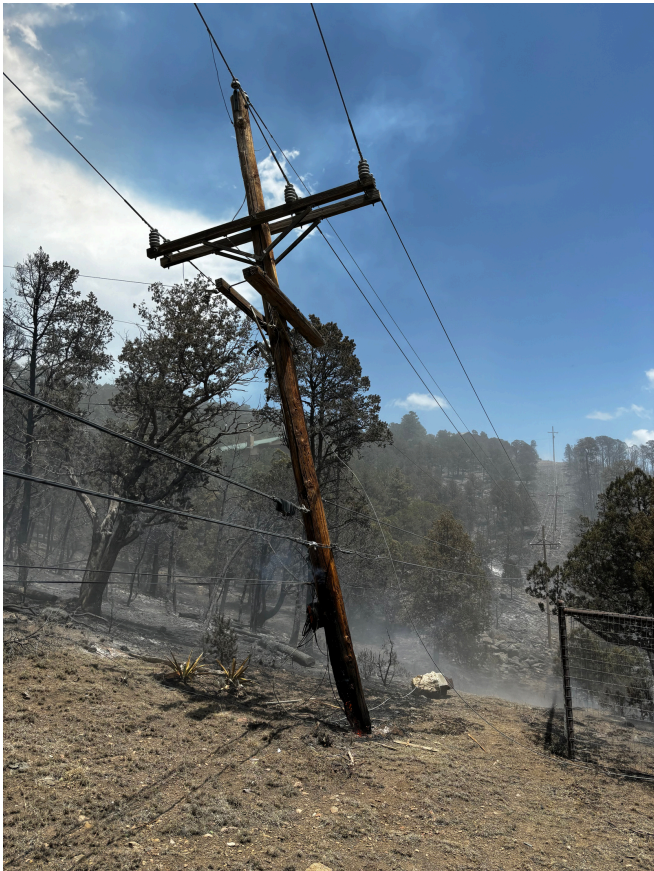
A sample of the damage to an electric pole from the South Fork Fire in Alto, highlighting the challenges faced by crews working to restore power. Over 80 poles replaced and 160 meters disconnected from the horrific incident.
